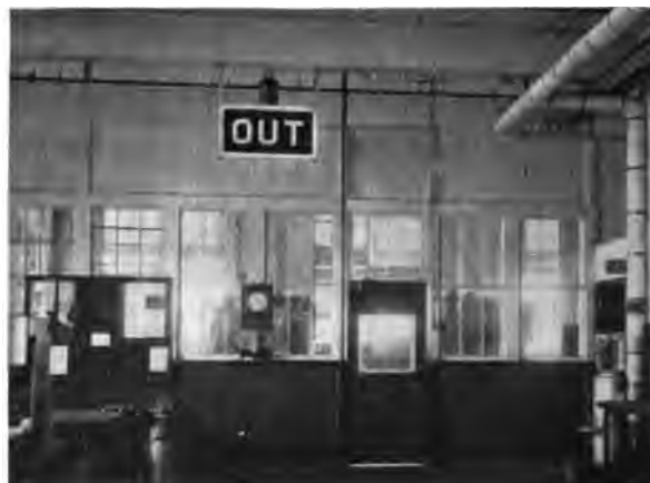
Fig. 4. "Out" Sign illuminated by Fire Alarm. (General Electric Co.)
